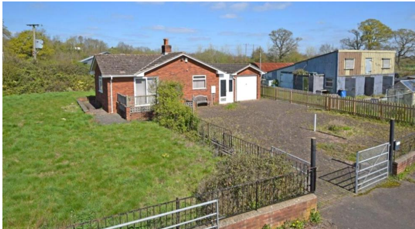
Looking west at the main buildings on the site, from Langaton Lane
